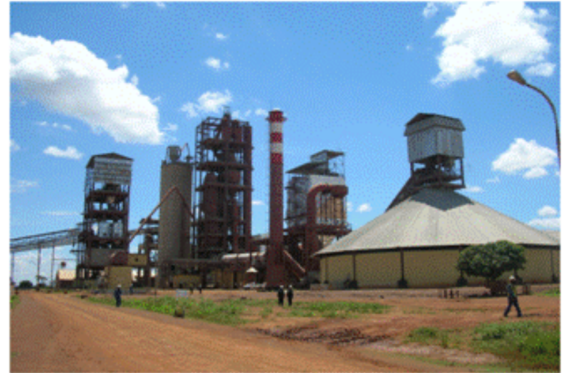
1000 TPD Cement plant for Zambezi Portland, Zambia( S. Africa)
