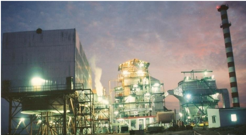
6.6 MW Municipal Waste Power Plant- EPC for Selco International , A.P ( India)
