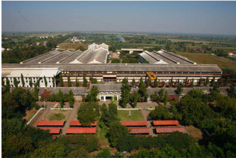
Heavy Engineering at Walchandnagar
