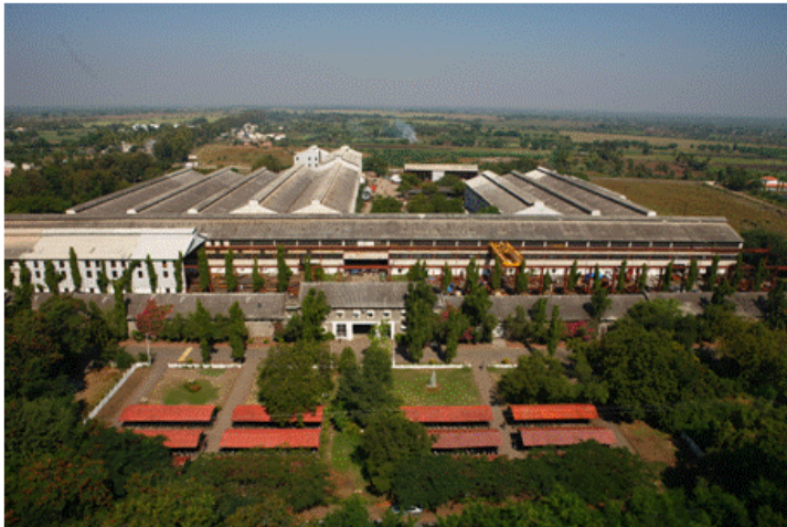
Aerial view of Walchandnagar plant
