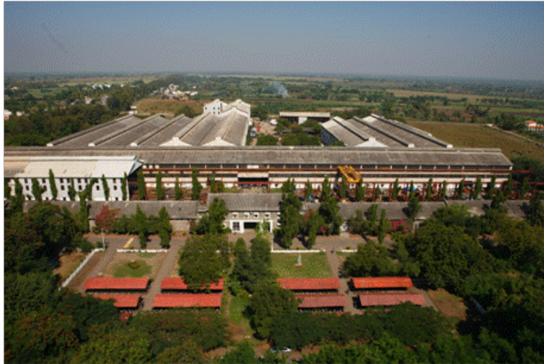
Heavy Engineering at Walchandnagar
