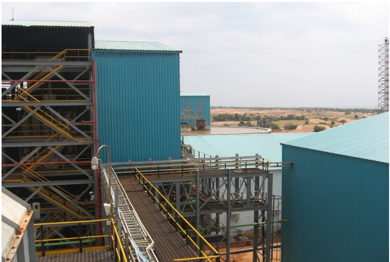
Pre-Concentration Plant Building
